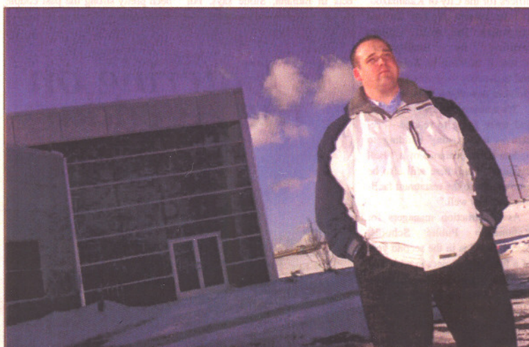
Dave Trombley of Maverick Construction Company outside the recently completed Fluid Process Equipment building in the WMU Business Technology & Research Park. Photo 2/03 by Tony Dugal.
